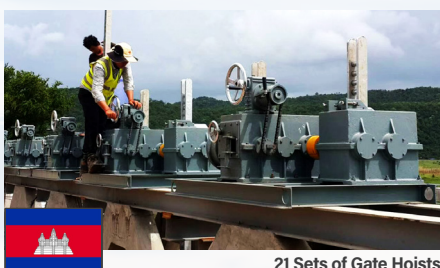
21 Sets of Gate Hoists
