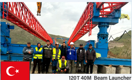
120T 40M Beam Launcher
