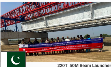
220T 50M Beam Launcher
